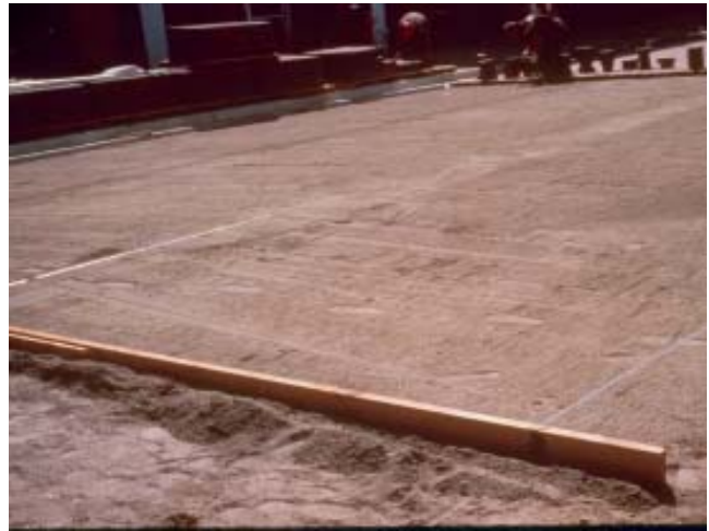
Figure 5—Screeded Bedding Sand
