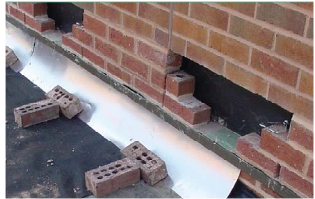
Photo 3 Flashing Installed in Alternating Sections
