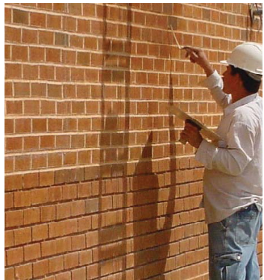
Photo 2 Repointing Mortar Joints
