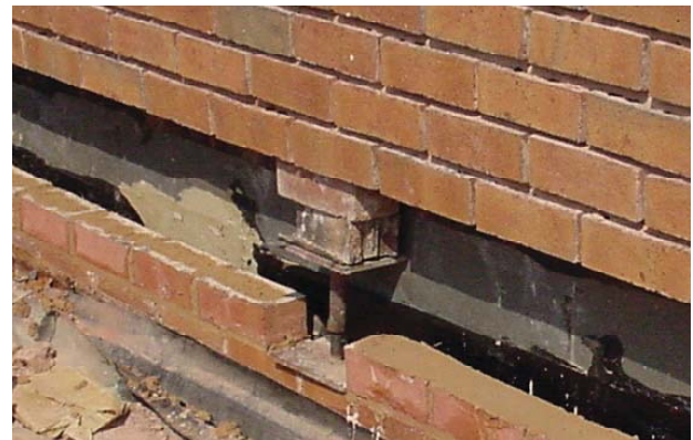
Photo 4 Flashing Installation Using Temporary Support
