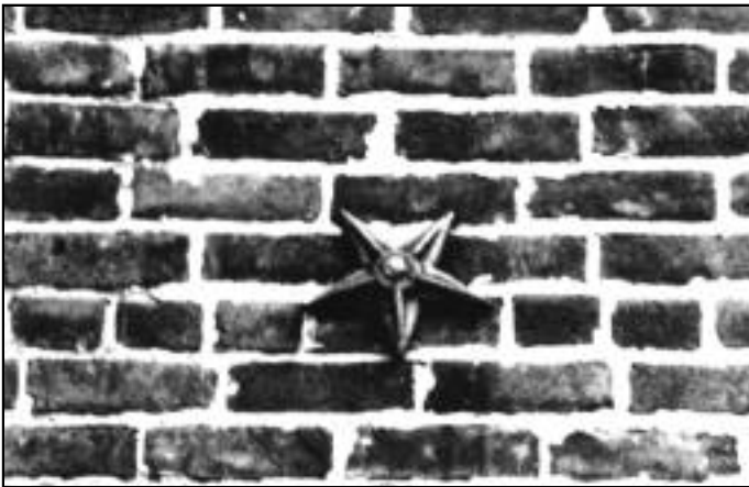
Decorative Through Bolt Bearing Plate FIG. 6
