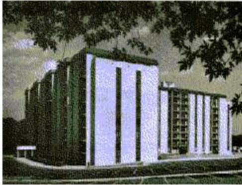
Woodlake Towers, Fairfax County, Virginia
