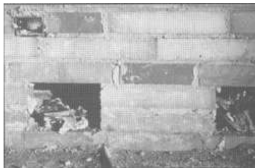
Example of Grout Space Cleanouts FIG. 1
