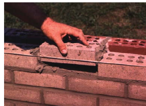
Photo 3 Placing the Closure
