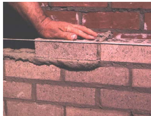
Photo 1 Shoving Brick into Place
